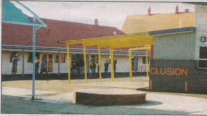
The redeveloped area at St Helens District High School.
