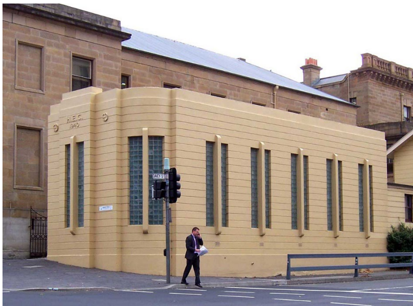
1940 - Hydro Electric Commission Sub Station, Davey Street, Hobart, Tasmania
