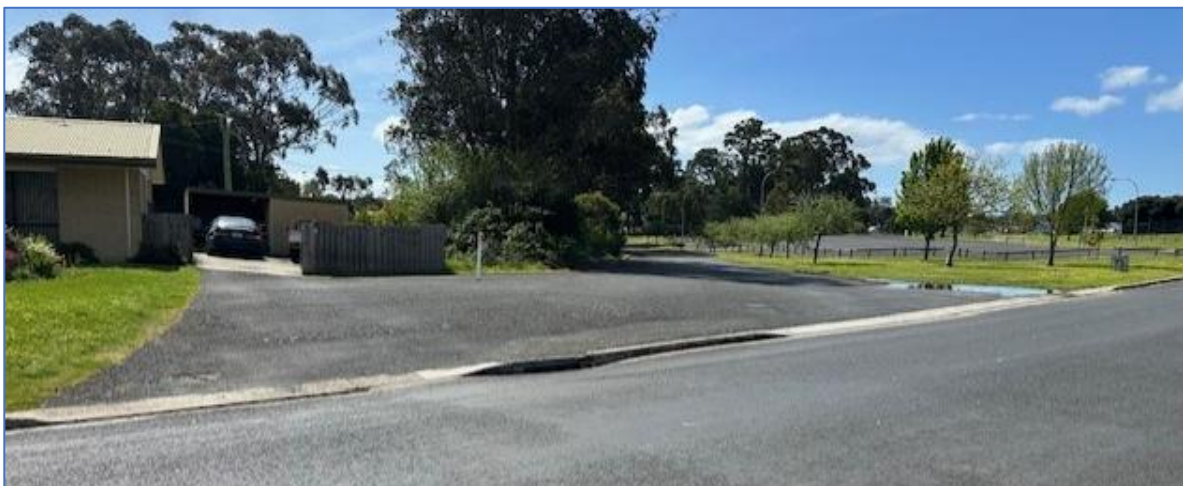
Photograph 4.6B – Accessway intersecting Bay Road including property driveway
