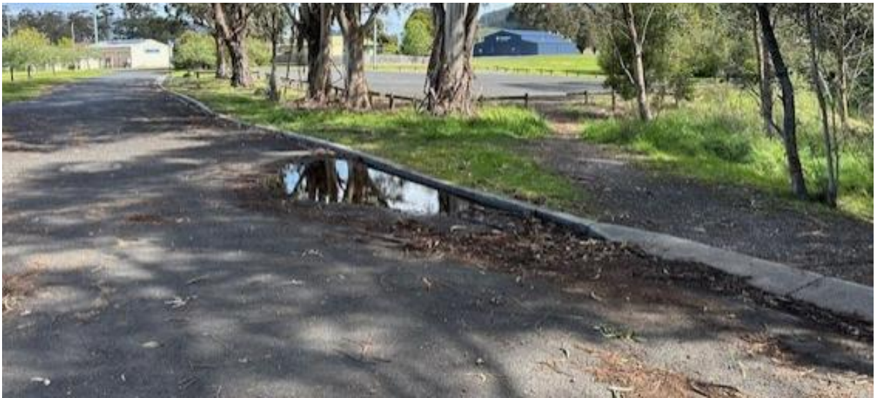
Photograph 8.0B – Water pooling at the Bay Drive access (eastern side)
