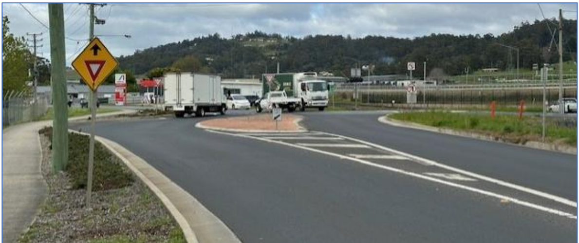
Photograph 4.5A – Available sight distance to the left (85 metres)
