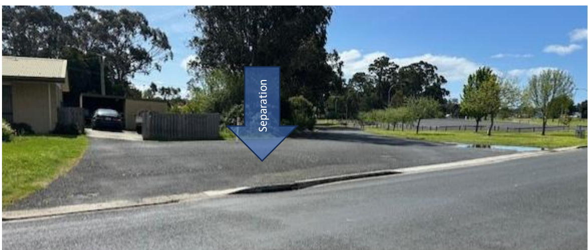
Photograph 8.2 – Access crossovers to Bay Drive
