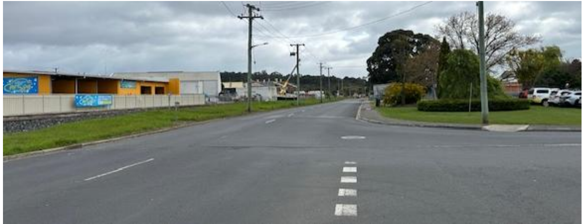
Photograph 4.2 – Devonport Road near Bay Road junction
