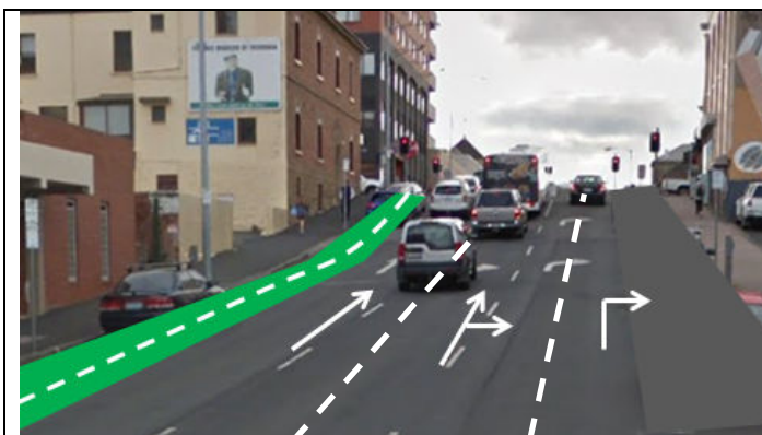
Less interruption to motor vehicle traffic and wider travel lanes if on-street parking was eliminated in this block between Davey & Macquarie.
