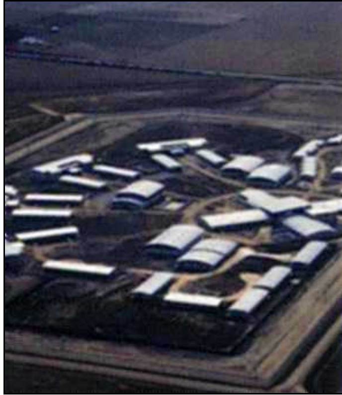
Aerial view of Fulham Correctional Centre
