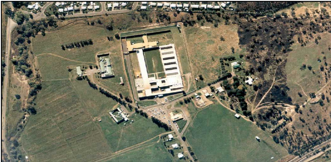
Aerial view of Risdon Prison
