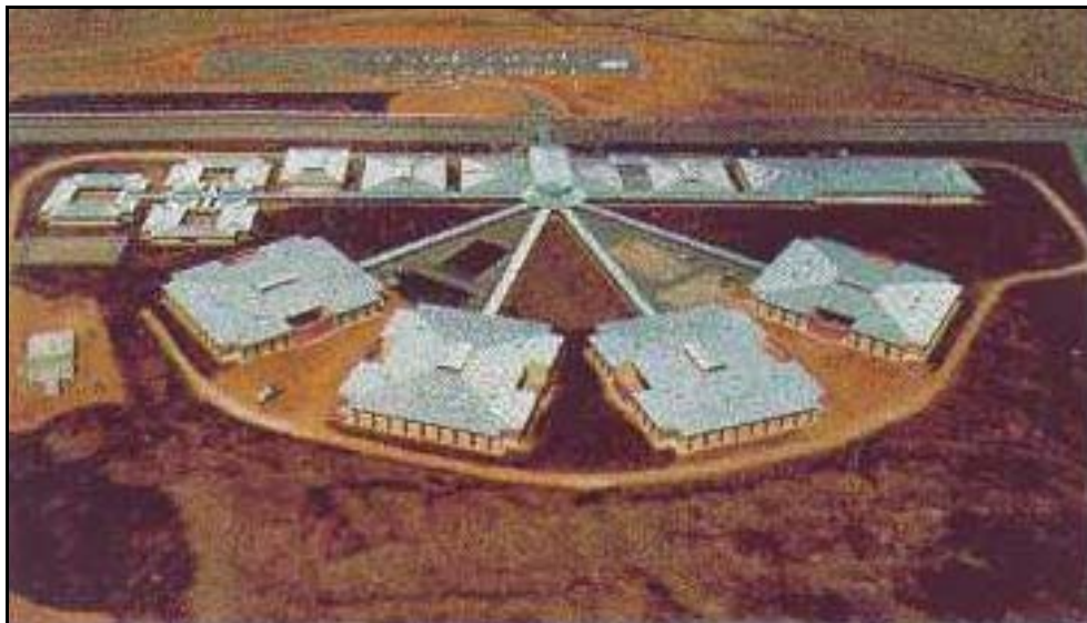
Aerial view of Junee Correctional Centre
