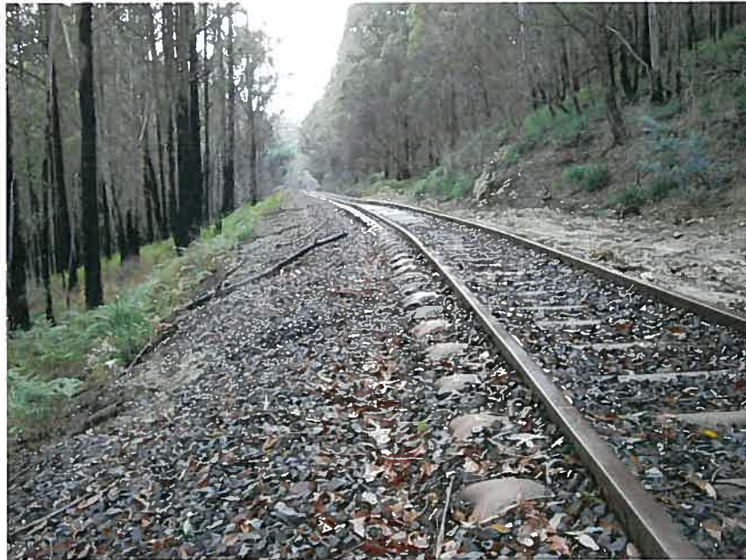
Typical condition steel sleepered track - Turners Marsh
