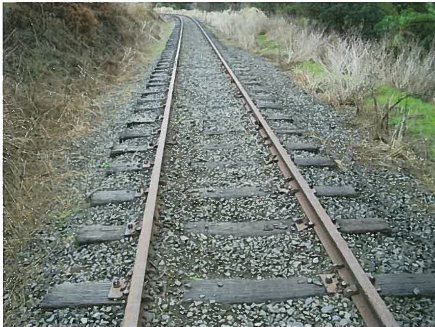
Typical condition of treated timber sleepered track - Lalla
