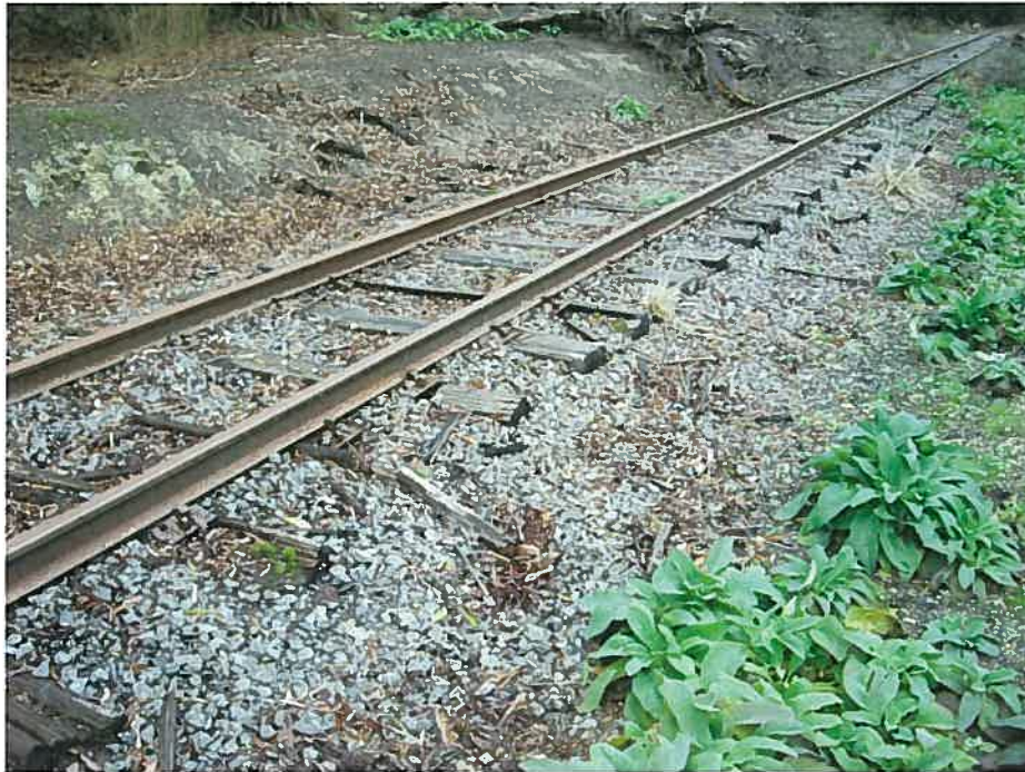
Typical condition non-treated timber sleepered track - Denison Gorge.
