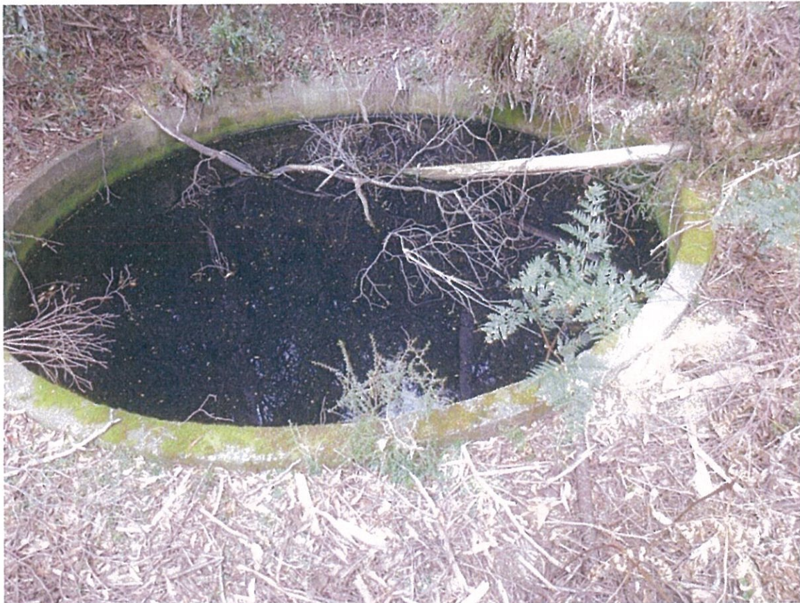
The tank that fed the standpipe.
