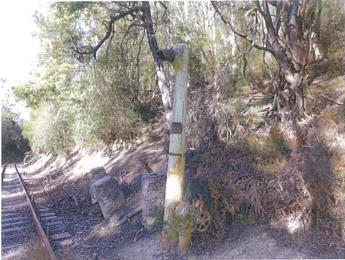
The standpipe that previously rewatered steam trains.
