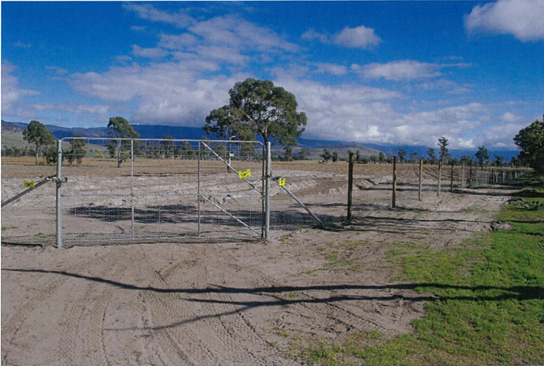
Image of deer proof fence to protect University of Tasmania plant trials on 'Connorville'. The fence cost $46,000 to protect a 17ha paddock. Several deer jumped over this fence and damaged the trials.
