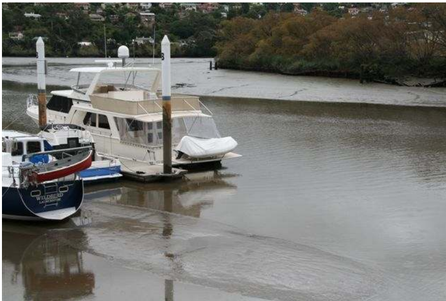
Another example of siltation narrowing the navigable channel
