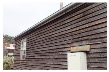
Figure 5: Fascia board at guttering
