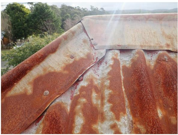
Figure 8: Evidence of paint noted in and around ridge capping
