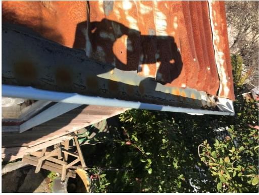
Figure 3: The gutters appeared to be new and clean
