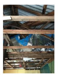
Figure 2: Timber roof framing in ceiling space
