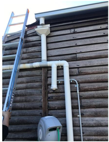
Figure 4: The water collection system. First flush systems were present on the downpipes
