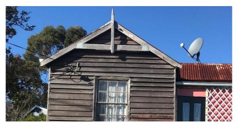
Figure 4: Barge boards on northern gable
