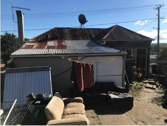
Figure 1: The roof was identified as corrugated iron, with no evidence of paint noted
