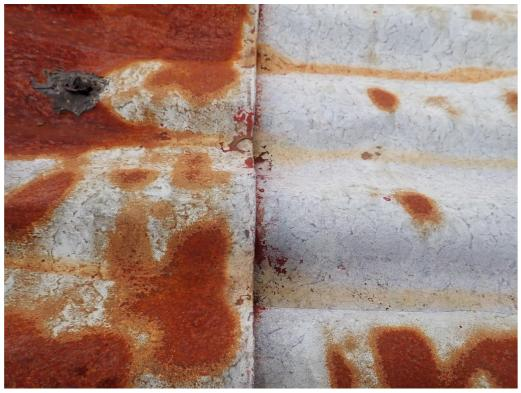
Figure 9: Small amounts of paint noted between some sheets
