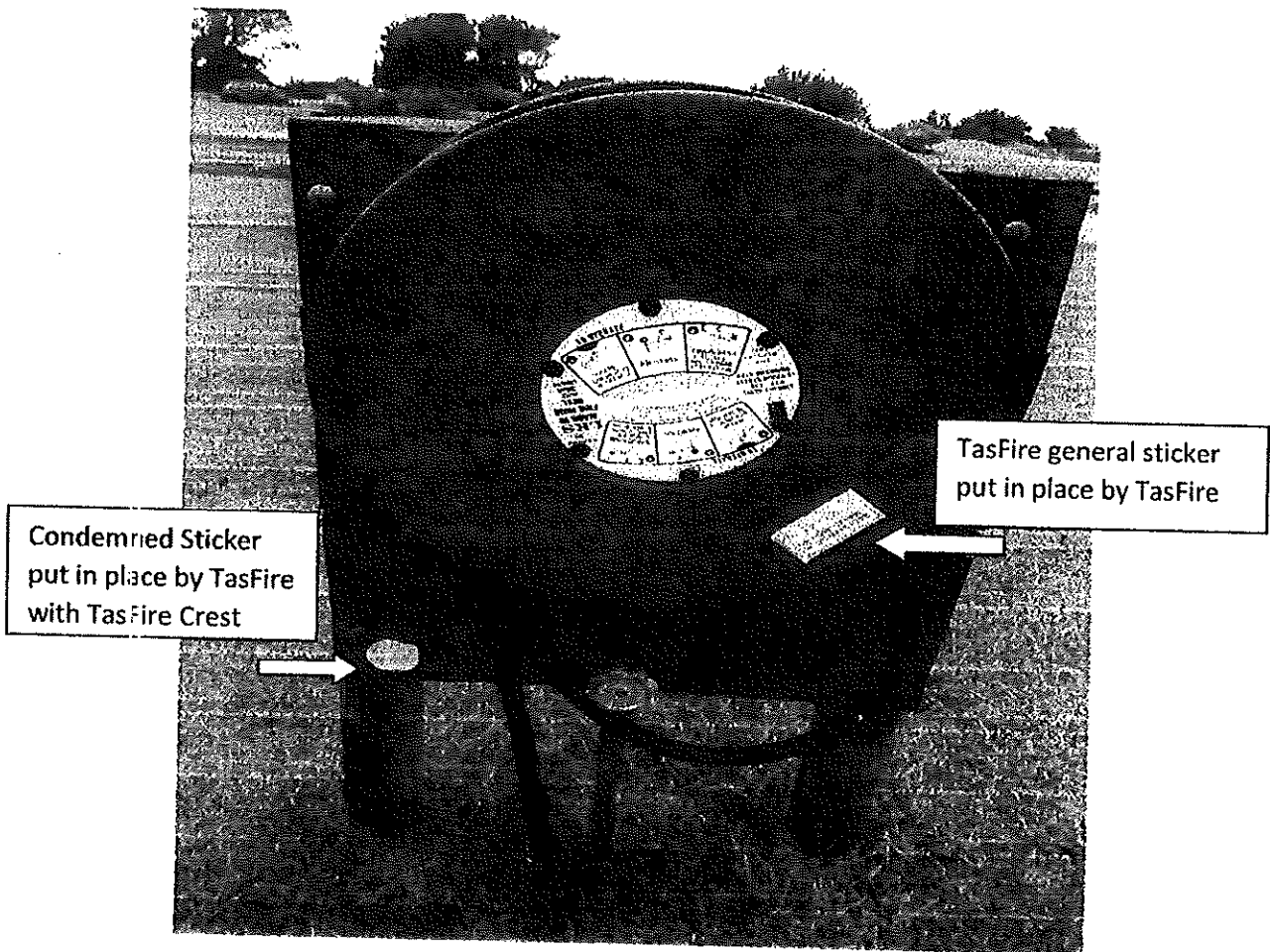
Image 1: Fire hose reel condemned by TasFire with all their own stickers placed on reel
