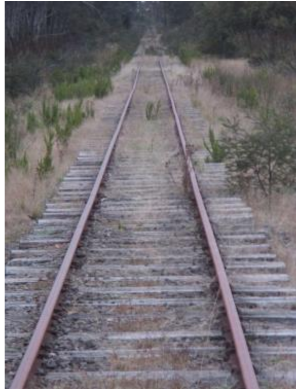
Below: Plated Timber sleepers through 400 m Radius curve
