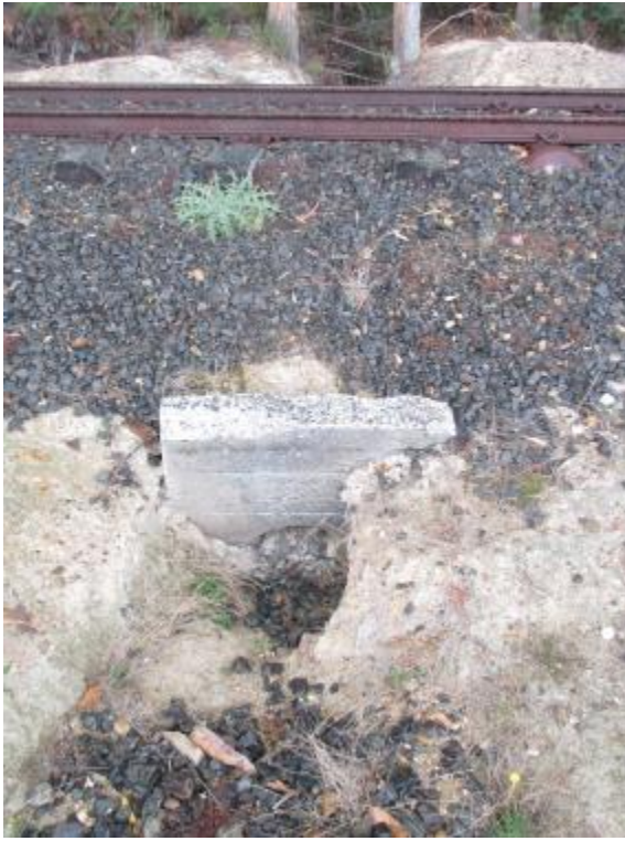
Below: Inlet blocked, Formation collapse 9249
