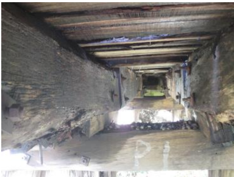
Below : Aging timber support beams; timber-packed onto trestle cross-beams.
