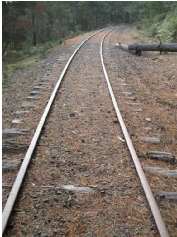
Unplated Timber sleepers through 160 m Radius curve.
