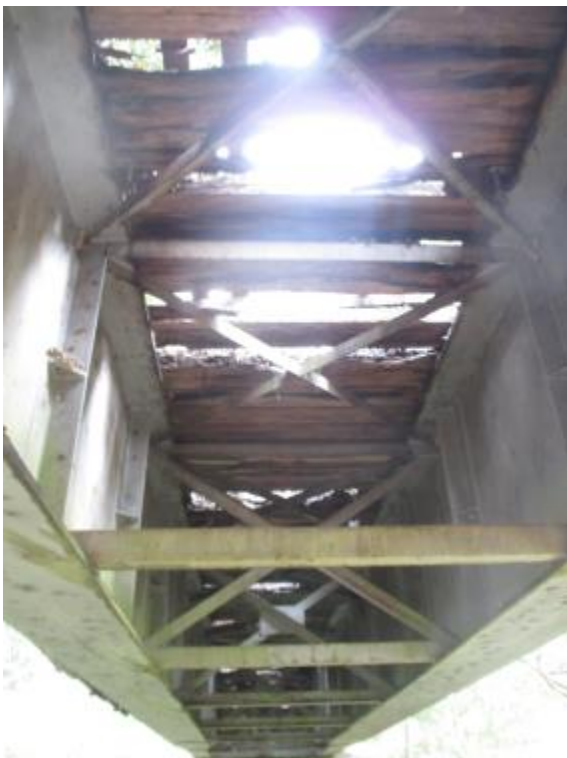
9089 Extensive failing of timber track-decking.
