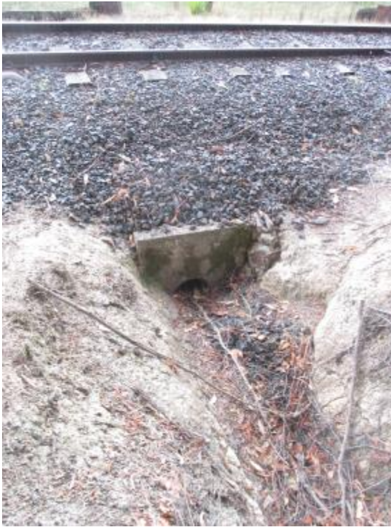
Below: Outlet h'wall by-passed by flow 9218
