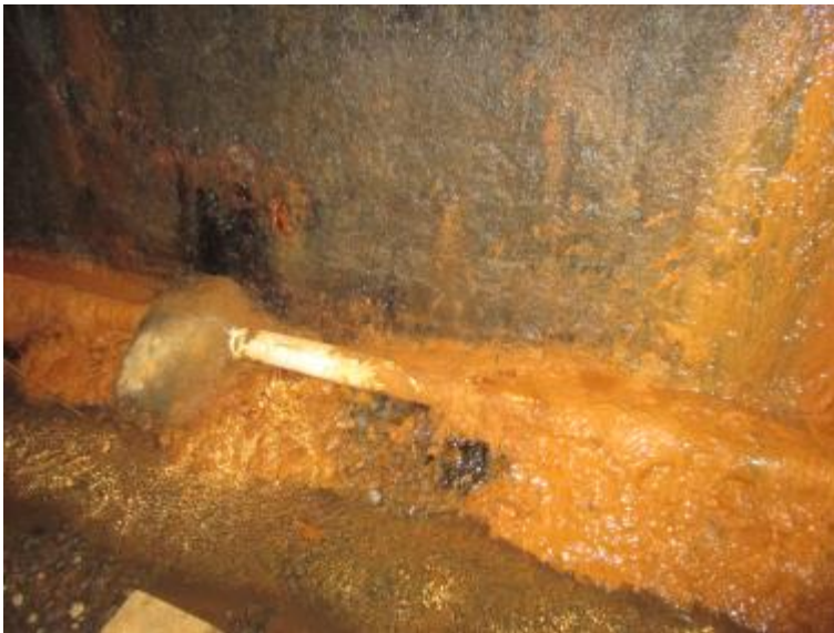
9549 'Spring' water weeping above 460 mm thick conc.
