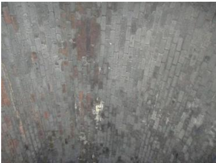
9551 Roof's Brick-lined Arch, 360 mm.
