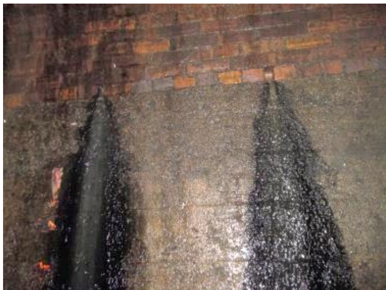
9541 Conc-to-Brick lining, at 2.4 m height.
