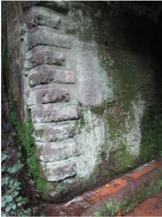
9597 Portal Pillars, 460 mm thick, in good condition.
