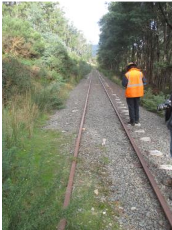
Unplated Timber sleepers in long Tangent.
