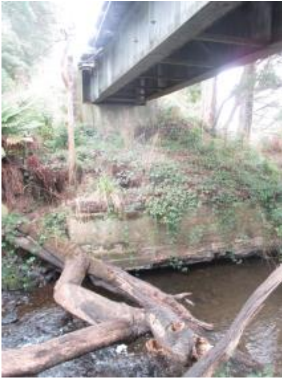
9095 Conc. abutment's apron slight under-cut.
