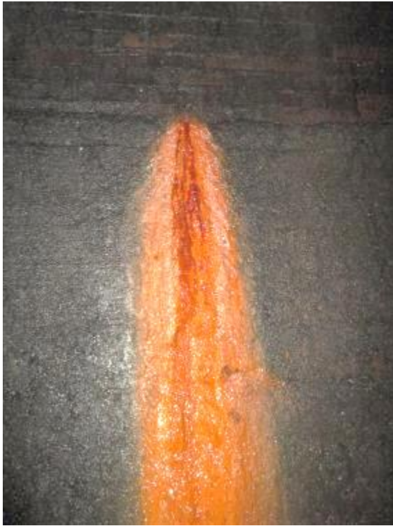
9549 'Spring' water weeping above 460 mm thick conc.
