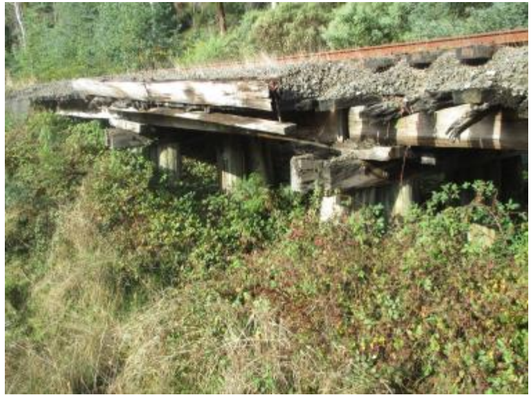
Below : Aging timber support beams; timber-packed onto trestle cross-beams.
