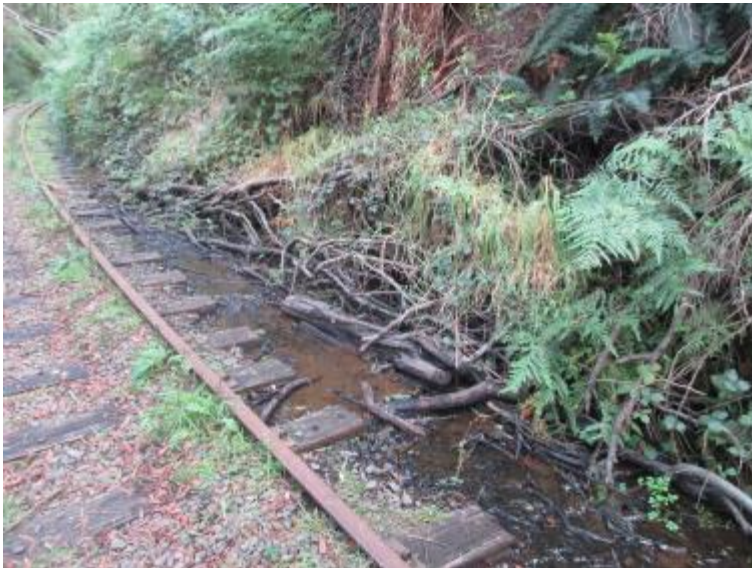
9575 Below : Vegetation invading side-drain, which is then invading the Track-skeleton.
