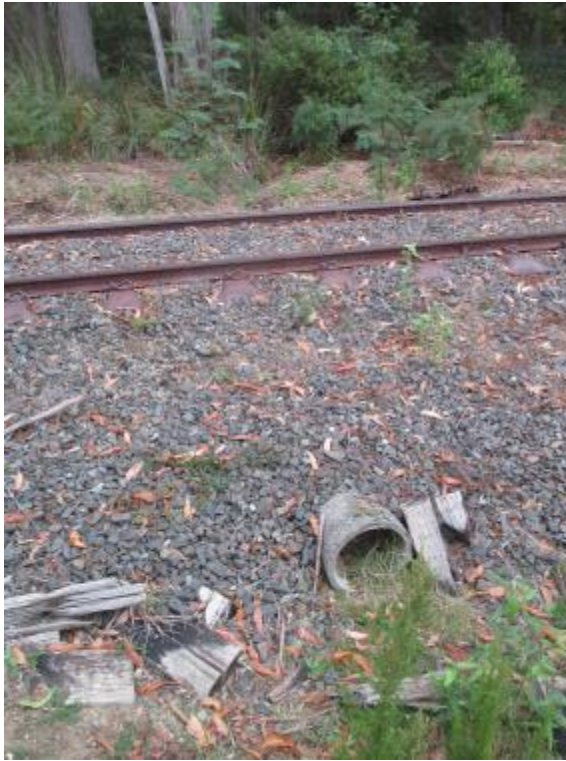
Below: Inlet damaged, partly ineffective. 8908
