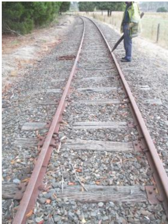
Below: Plated Timber sleepers through 400 m Radius curve
