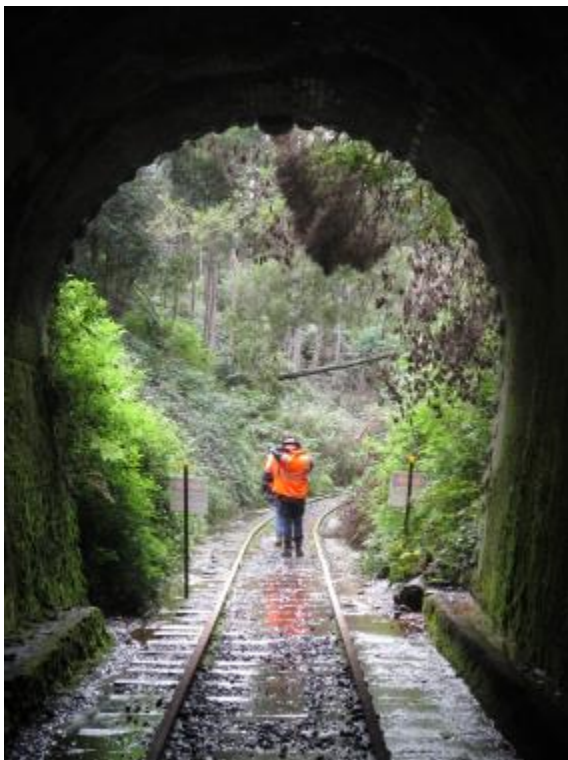
9539 To achieve vertical clearance to roof-arch, a small number of steel sleepers have been used over a section of extra-hard rock floor.
