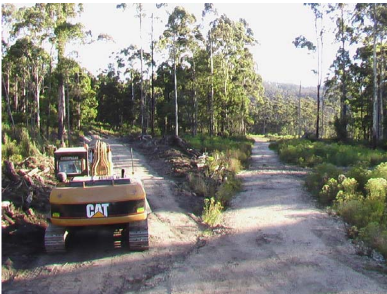
The new road (left) under construction.
