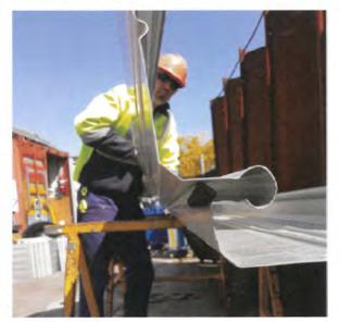
The sheet shown in the photo above is not properly engaged. The over needs to cover the under completely with the edge of the over touching the vertical face of the previous sheet.
