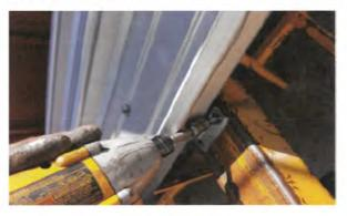
FreeForm<sup>™</sup> fixing clips are screwed into the purlins oriented to allow for the desired direction of the ribs.
