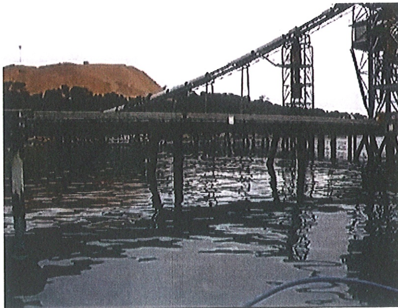
Photo shows the trestle beams that span from each concrete wharf head dolphin
