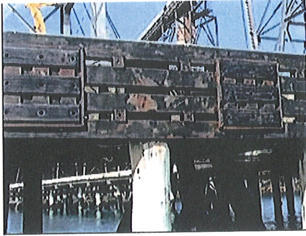
Photo shows the wharf face fender frames and corrosion
