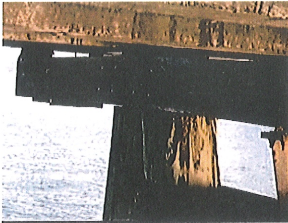
Photo shows the severity of the cracked crossheads
