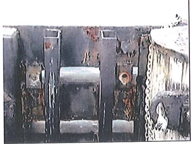
Photo shows the wharf face fender frames and corrosion
