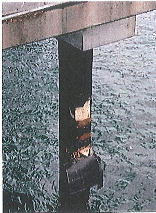
Photo shows the condition of some of the pile wrapping
