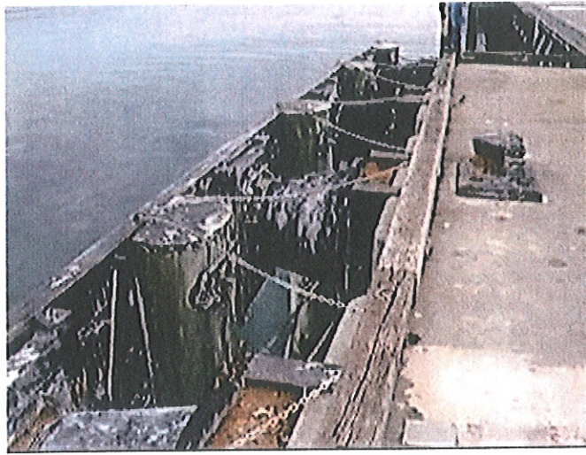
Photo shows the fender system configuration
