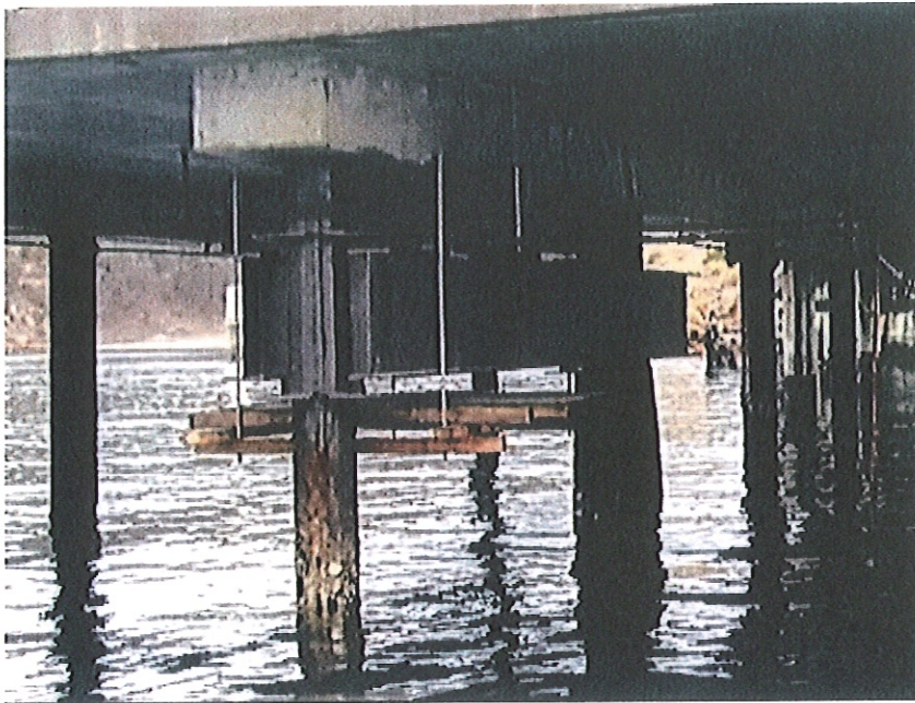
Photo shows the attempt to support the decaying concrete beams
