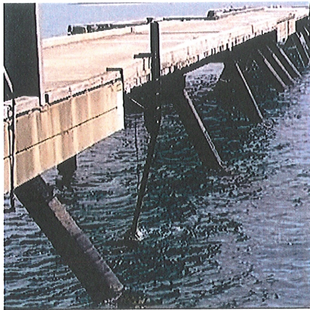
Photo shows damaged non-compliant safety ladders
