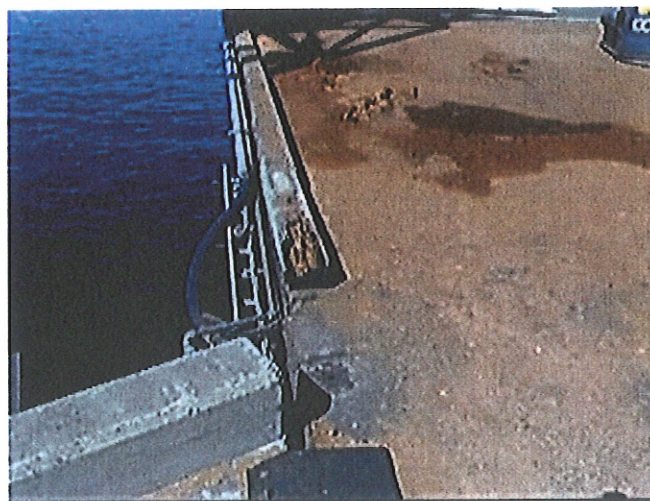
Photo shows damaged deteriorated wharf curb sections
