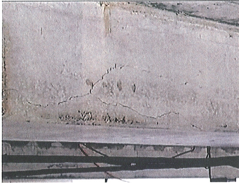
Photo shows the severity of the cracking to the main beams in the concrete wharf head
