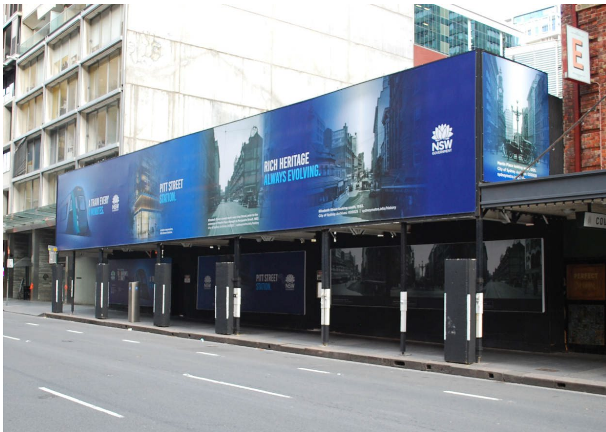
Figure 6b shows an example of “B” class hoarding (10kPa rating) overhead protection proposed over part of Davey Street
