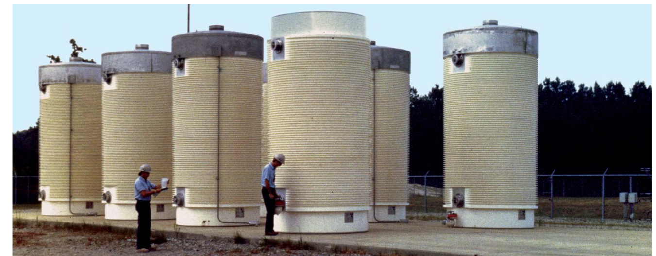
Fig 3: Spent fuel in dry store casks (USA)Spent fuel reprocessing
