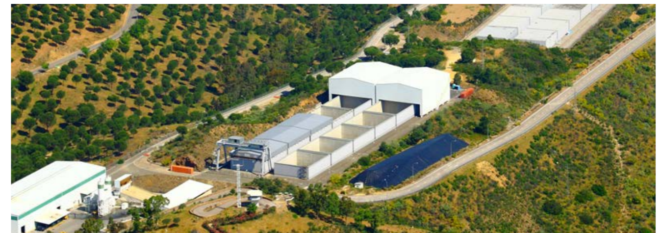
Fig 1: El Cabril Disposal Facility, Cordoba, Andalusia, Spain (ENRESA)
