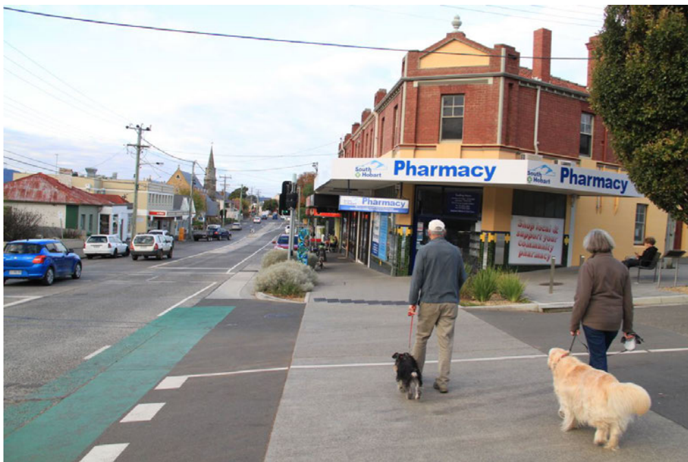
Elboden St and Macquarie St junction “raised threshold” treatment - constructed 2019.
