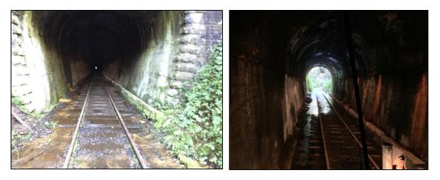
Figure 20. – Pictures of tunnel showing failed drainage system and flooded track
