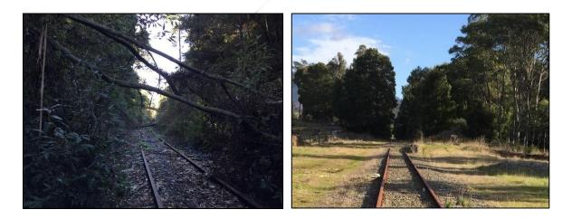
Figure 22. – Examples of areas requiring vegetation clearing
