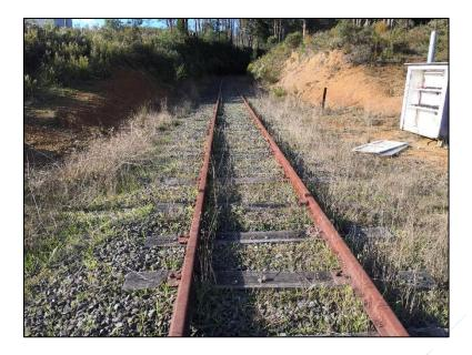
Figure 21. – Picture of silted cess drains
