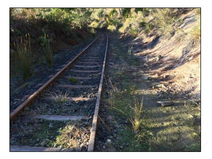
Figure 6. – Example of a silted cess drain
