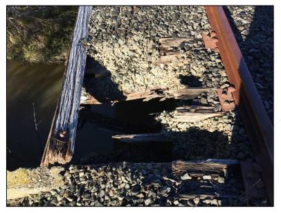
Figure 12. – Picture of a collapsing bridge deck - typical of many bridge decks on the North East line
