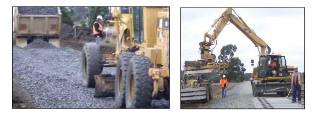
Figure 9. - Showing some of the work involved in rebuilding a level crossing
