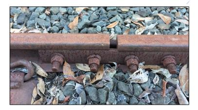
Figure 1. – Rusted fishplate
