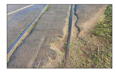
Figure 7. – Deteriorated level crossing at Scottsdale
