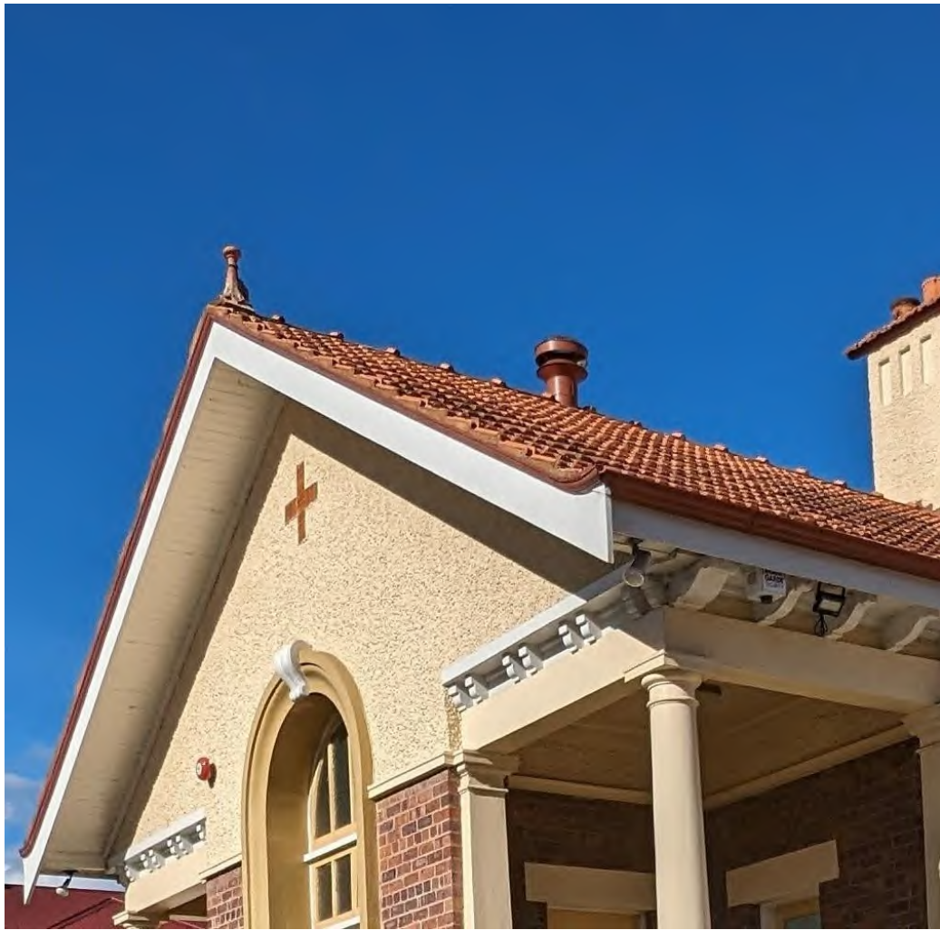
MATERIALITY & DETAILING: STUCCO, TERRACOTTA TILES, TIMBER DETAILING, RED BRICK, CURVED / ARCHED WINDOW. COLUMNS
