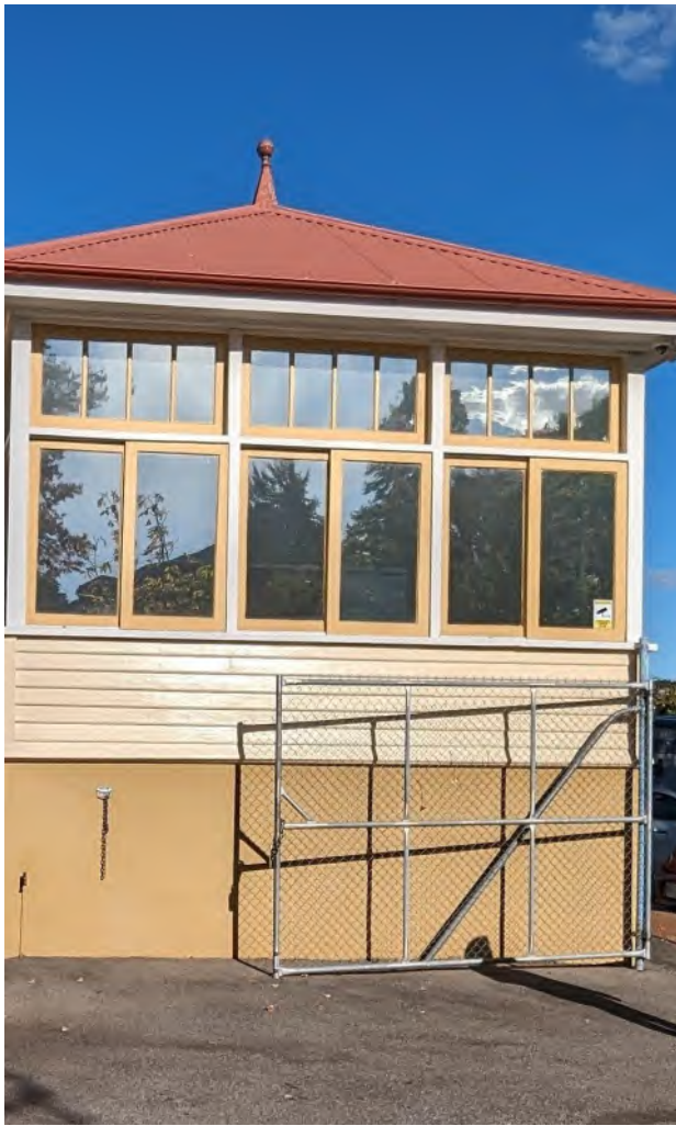
MATERIALITY & FORM: FOUR 'TURRETS' ARE PLACED AT THE FOUR CORNERS OF THE BUILDING, ANCHORING IT IN THE LANDSCAPE. THESE TURRETS ORIGINALLY ACTED AS SUN / DAY ROOMS. RENDERED BRICK, WEATHERBOARDS, CORRUGATED IRON ROOF.
