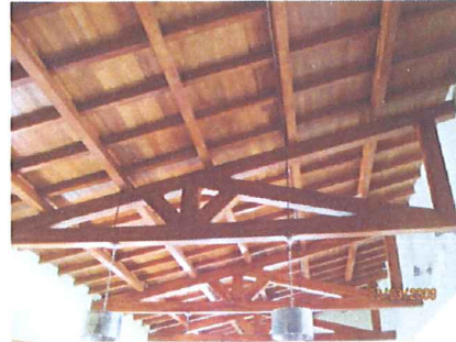
Figure 23: Interior ceiling of Villapol family meeting house showing use of globulus timber and laminated beams. (Photo T. Jaeger)
