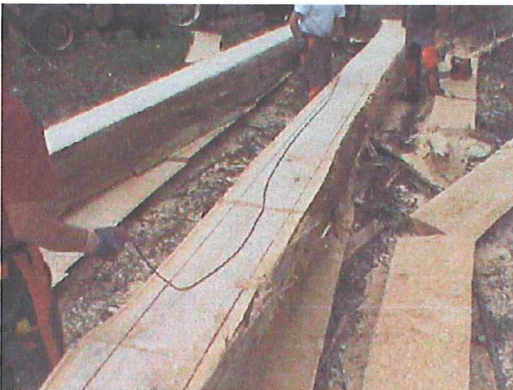
Figure 18: Preparing a log for cutting into a large beam.
