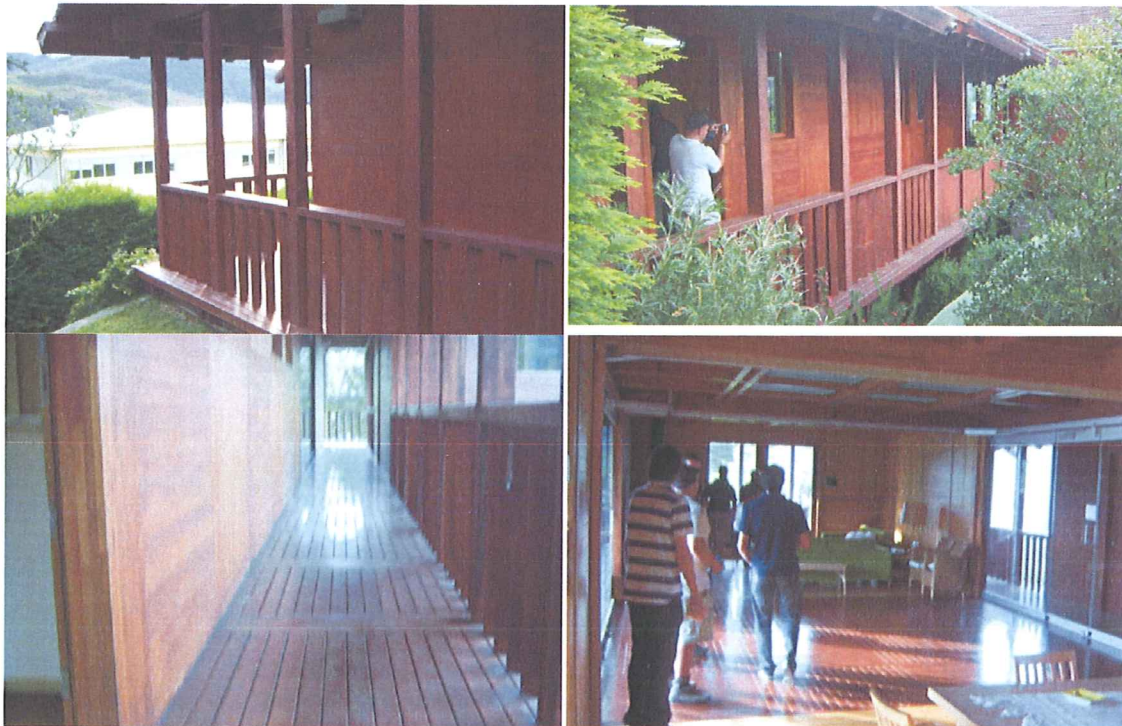
Figure 34: Various views of Villapol family demonstration house built entirely from Eucalyptus globulus (30,000 pieces of timber with no nails). (Photos P. Volker)
