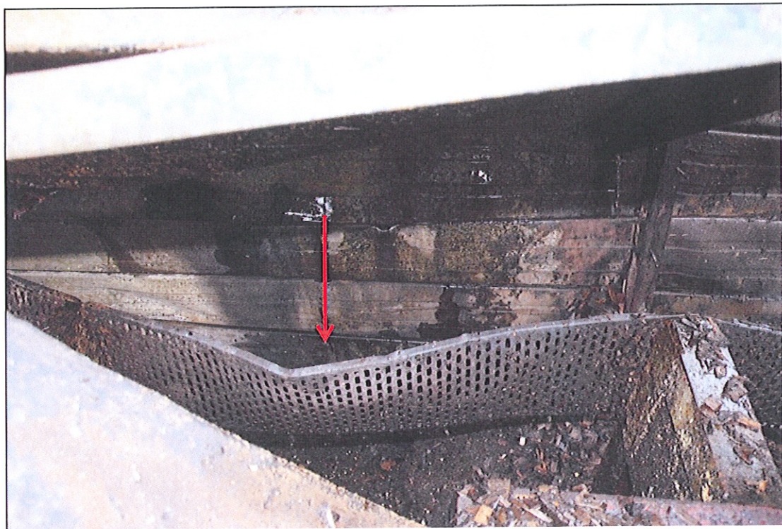
PHOTOGRAPH: 4. Lowest point of heat damage to retaining wall
