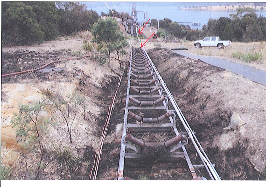
PHOTOGRAPH: 7. Area of removed conveyor belt frame.
