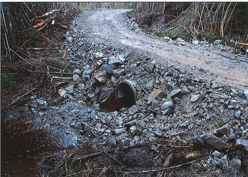
Well constructed concrete pipe culvert.
