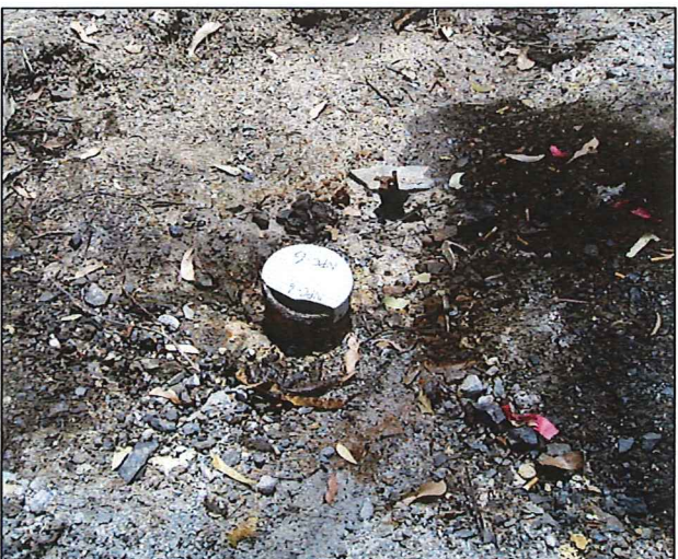
Broken PVC cap on steel collar.
