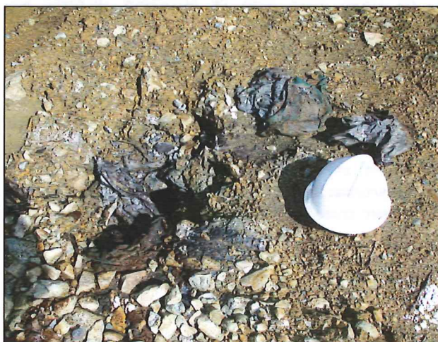
Open hole jammed with grease-soaked rags.
