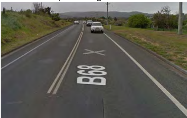
Fig10. 1287 Channel Highway, Northbound
