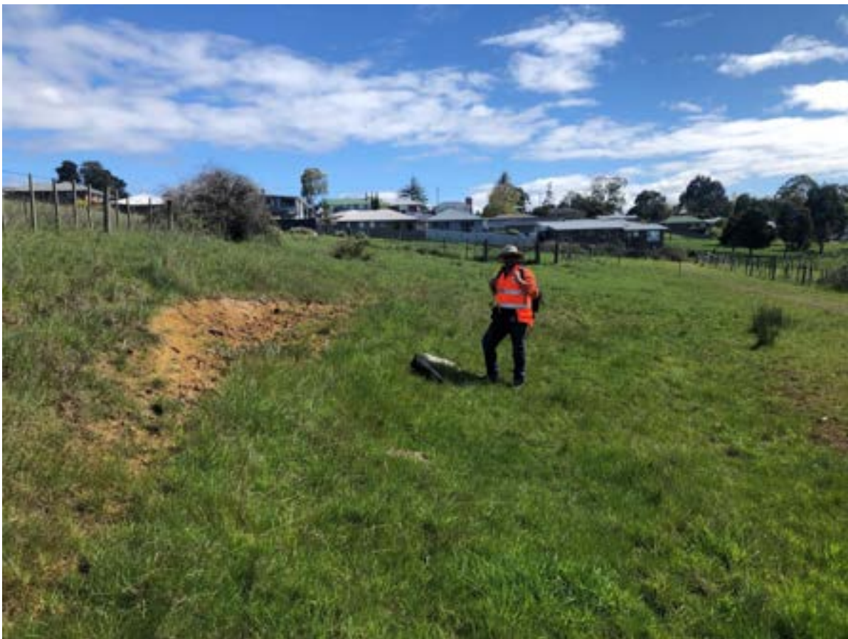
Figure 3-4 Historical cut batter exposing Launceston Group sediments. Adjacent to access track in north portion of site
