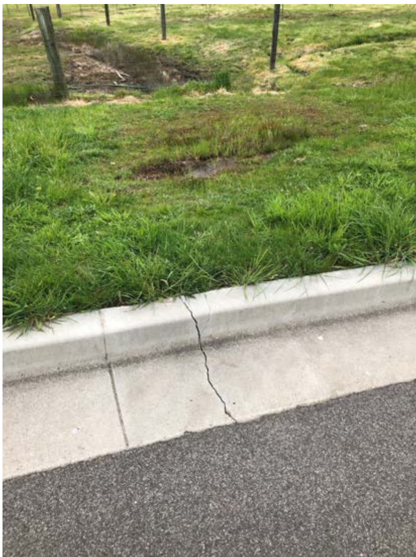
Figure 3-14 Cracking through kerb in new road south of site
